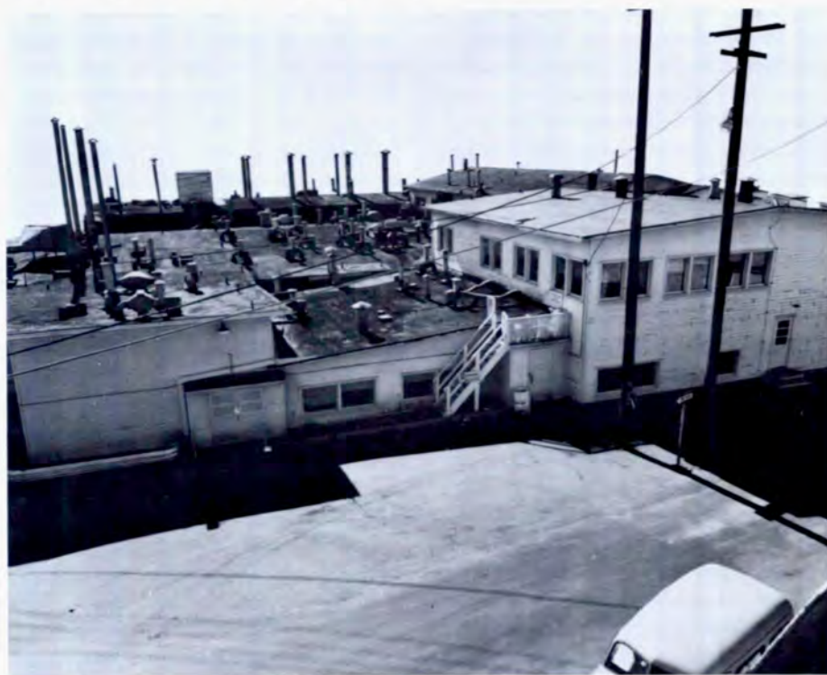
D Building, the air-conditioned wartime plutonium laboratory, bristling with separate external vents.
